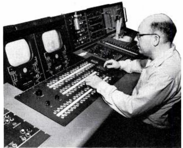
WKRC installation includes new RCA transistor switching and special effects system
